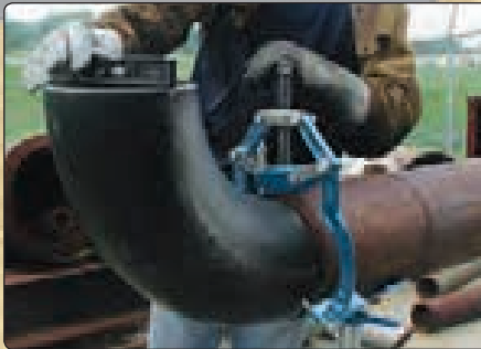
The E-Z Fit Clamp works great for holding fittings in position for welding.
